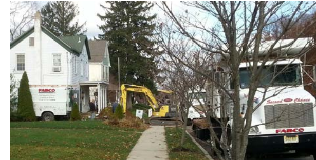
Underground Storage Tank Removal
