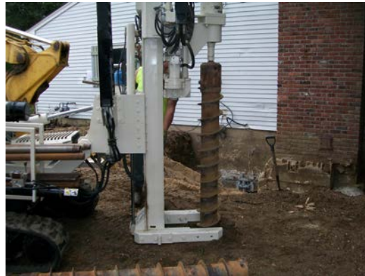
Groundwater Monitor Well Installation
